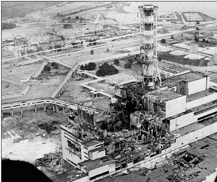
Figure 2. Chernobyl nuclear power plant shortly after the accident on 26 April 1986.
