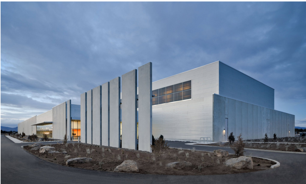
Figure 3.9: Brand new (April 15 th , 2011) Facebook's data centre in Prineville, Oregon. It received LEED (Leadership in Energy and Environmental Design) Gold Certification on November 17 th , 2011, since it requires 52% less energy to operate than a comparable facility built to code requirement
