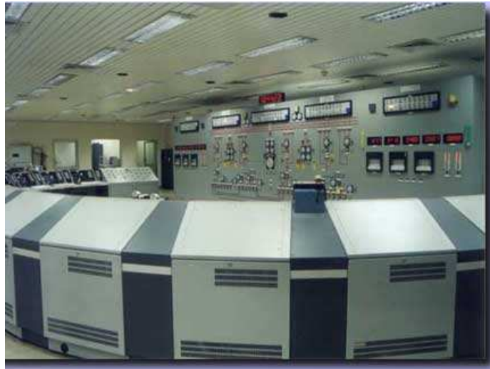
Figure 8: An analog control room.
