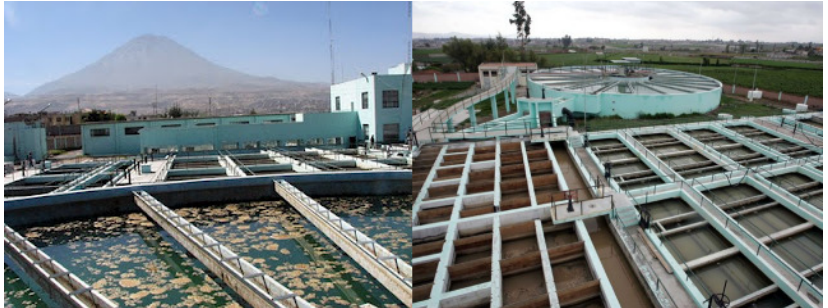
Figure: Drinking Water Plant La Tomilla, Arequipa - Peru
